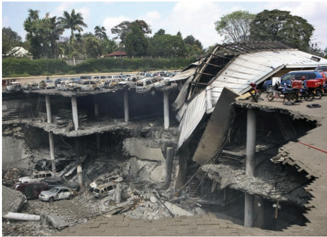
The collapse of three floors of Nairobi's Westgate Mall during the terrorist siege in 2013
